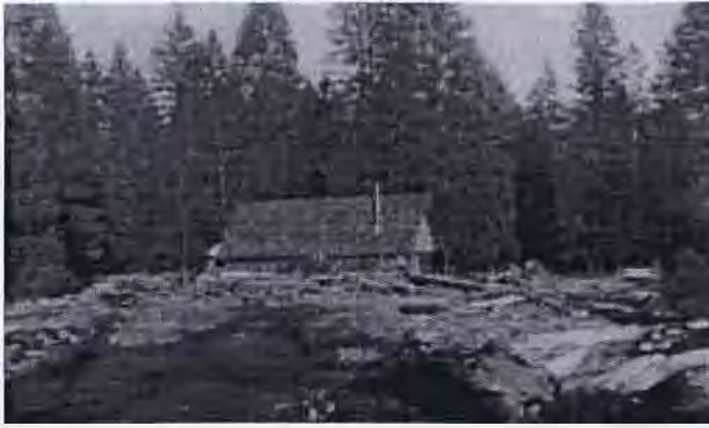
Coffee Creek Church with logs piled against it after the 1964 flood
