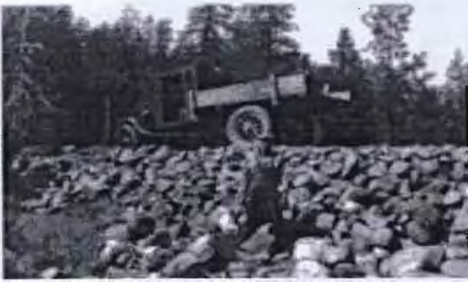
Frank Trumble Building the Dike for the Ponds
